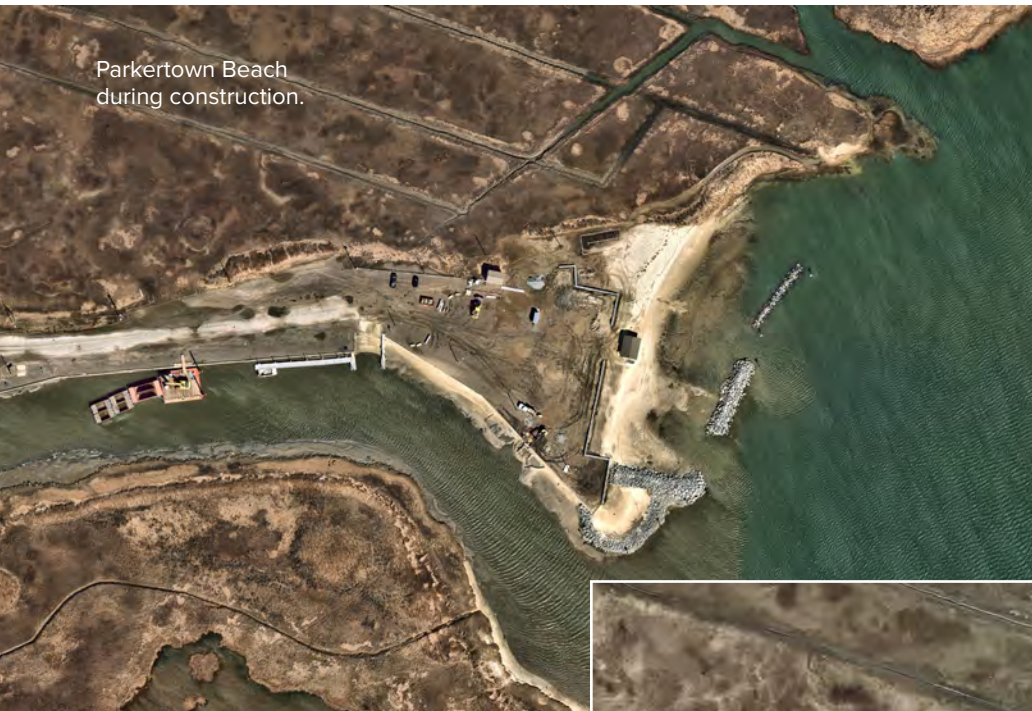
Parkertown Beach pre-construction.
