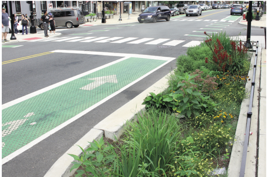
New environmentally friendly rain gardens beautify the streetscape while diverting excess stormwater from the sewer system. (Photo courtesy of T&M Associates)
